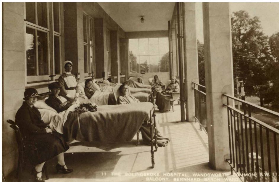
Bolingbroke Hospital balcony, Bernhard Baron ward, Patrick Loobey Collection, undated
